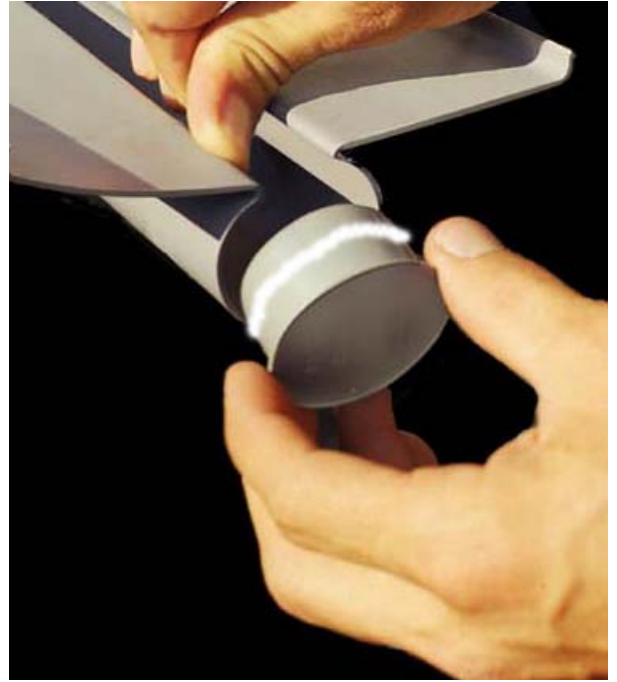
Silicon Beading around the Gutter Cap
